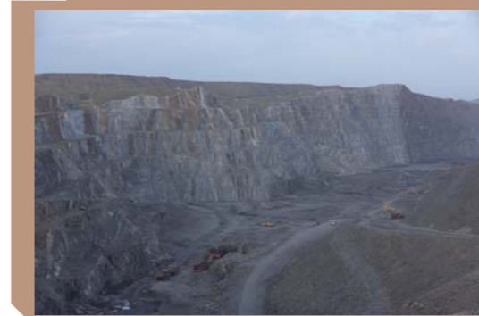
Neat mine slope
