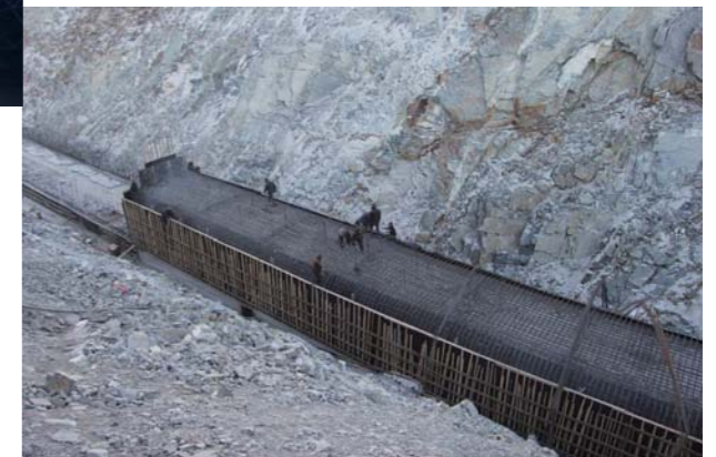
● No. 1 belt conveyor in Phase II expansion construction
