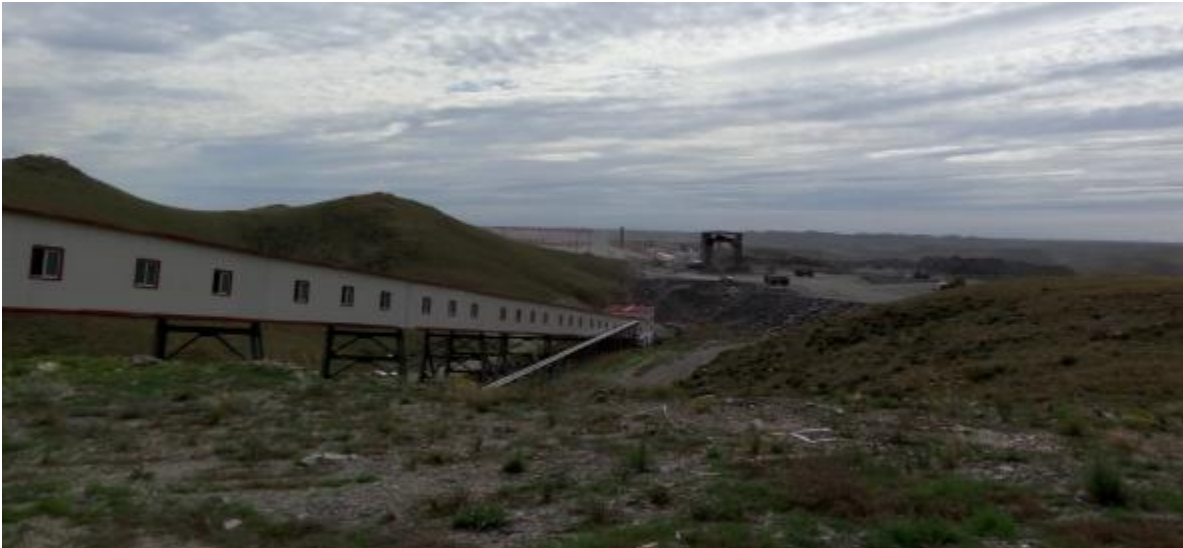
Figure 17-5: Photo of Phase 2 Crushing Station
