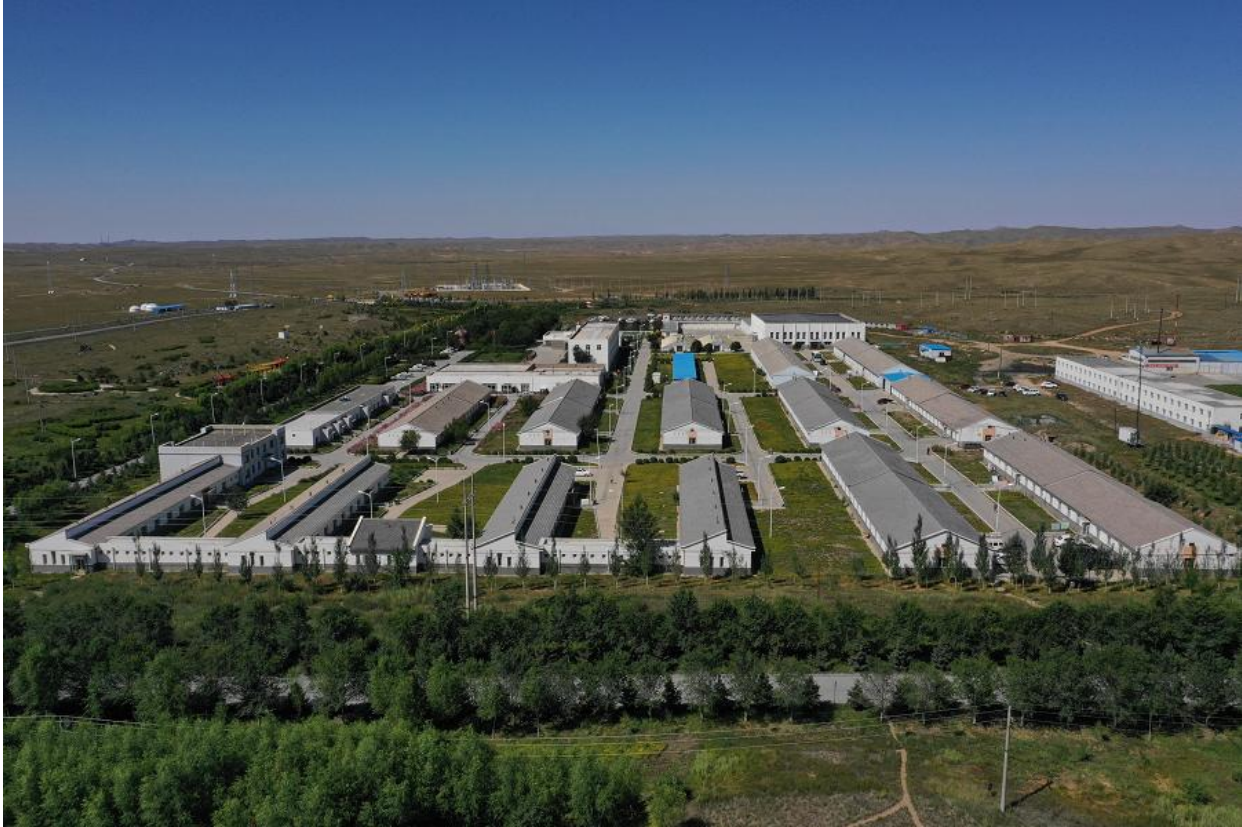
Figure 18-2: Photo of Staff Dormitory on Site
