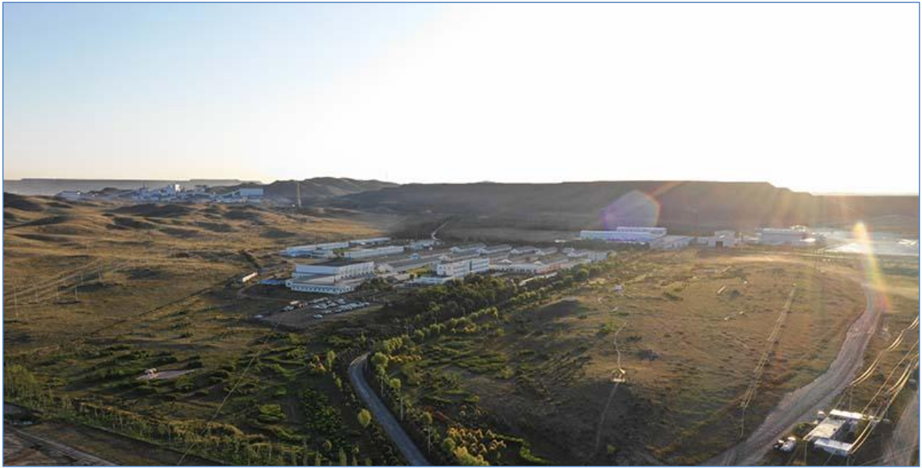
Figure 5- 1: Landscape in the Project Area (Looking North)
