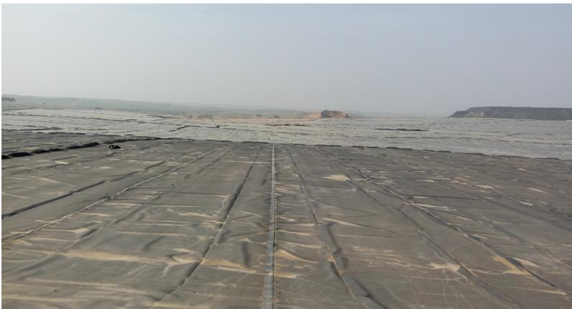
Figure 17-6: Photo of Phase 2 Heap Leach Pad
